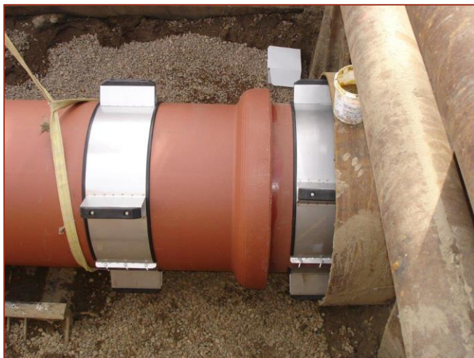
Fig 2: Stainless Steel Casing Spacers with polyethylene runners designed for a 30-inch Bell and Spigot VCP Pipe.
