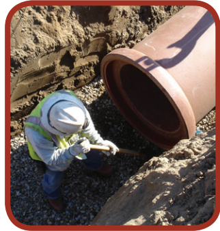
Figure 22: Constructing a bell hole during pipe laying
