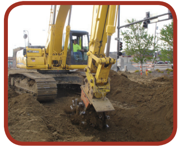
Figure 27: Hoe mounted sheepfoot roller compacting final backfill
