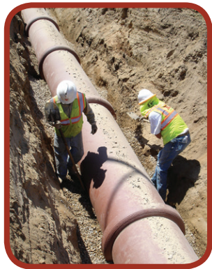
Figure 26: Shovel slicing the pipe haunches
