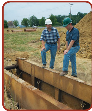
Figure 2: Inspectors are a vital link between specification and construction.
