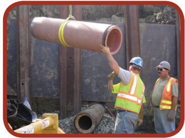
Figure 1: Lowering VCP Jacking pipe into the pit
