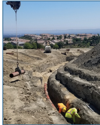
Figure 32: Installation of a curvilinear sewer
