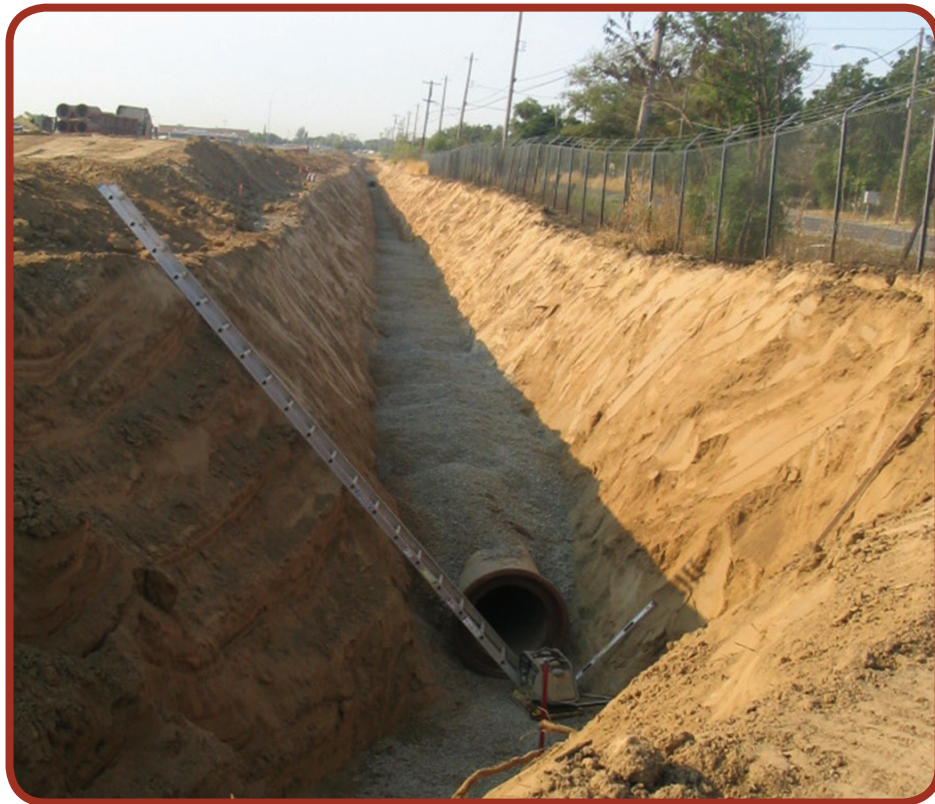
Figure 5-1: 30-inch pipe installed in a vee trench in Linda, CA.
