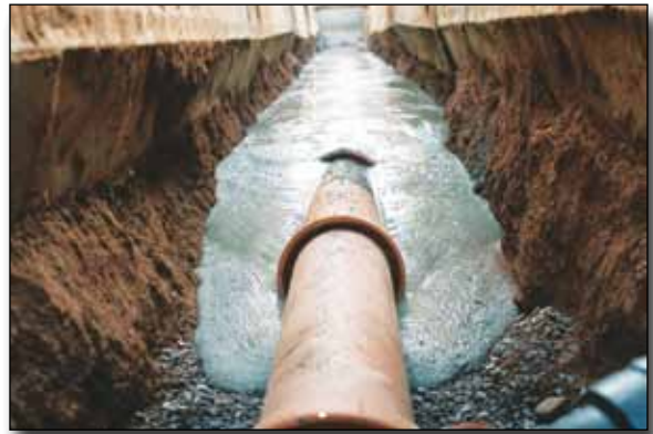
CLSM in the trench
