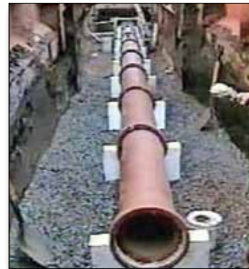
Foam block in trench
