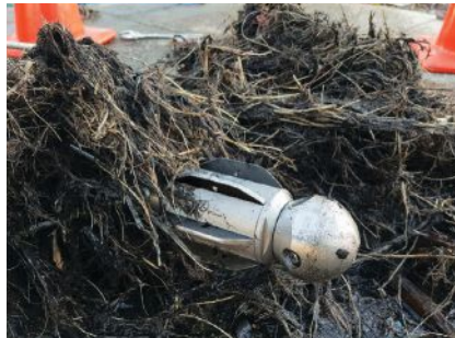
Rotational nozzles can be used to dislodge fibrous roots.
