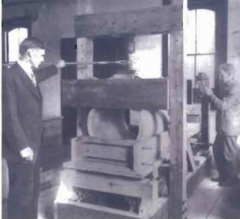
Professor Anson Marston Observing Early Pipe Tests at the Engineering Experiment Station, Ames, Iowa.
