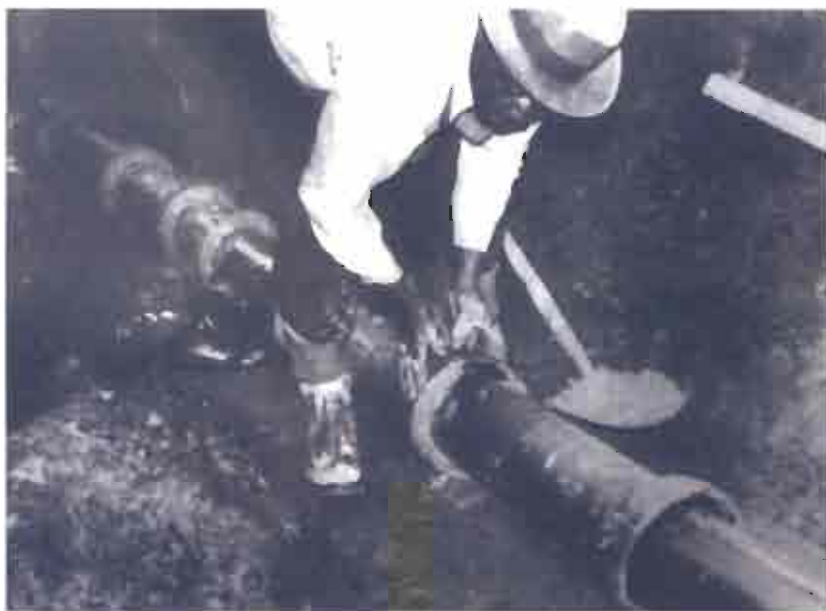
Top to bottom: Early Hot-Pour Field Joints and Early Cement Mortar Field Joints
