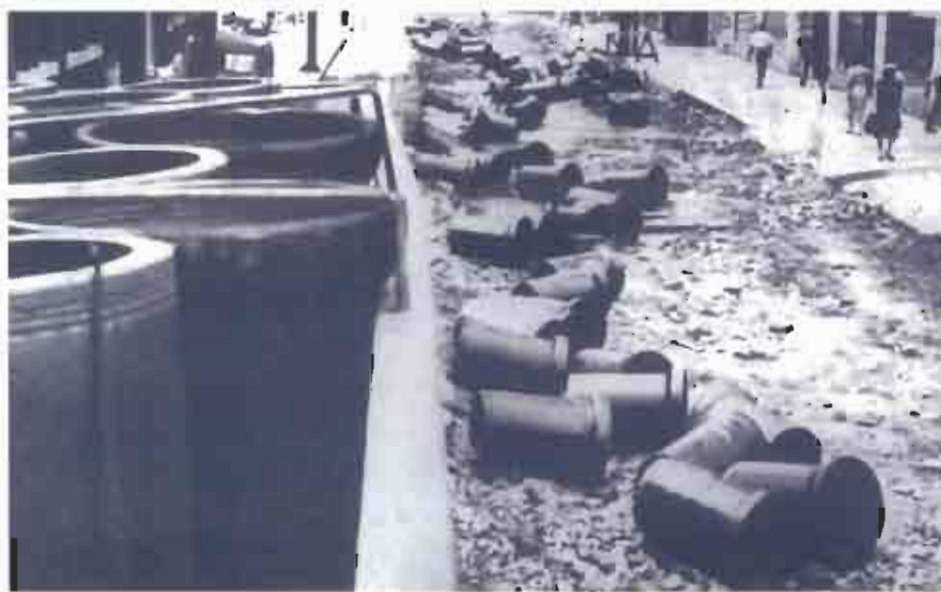
Early Clay Pipes Were Supplied Without Joints
