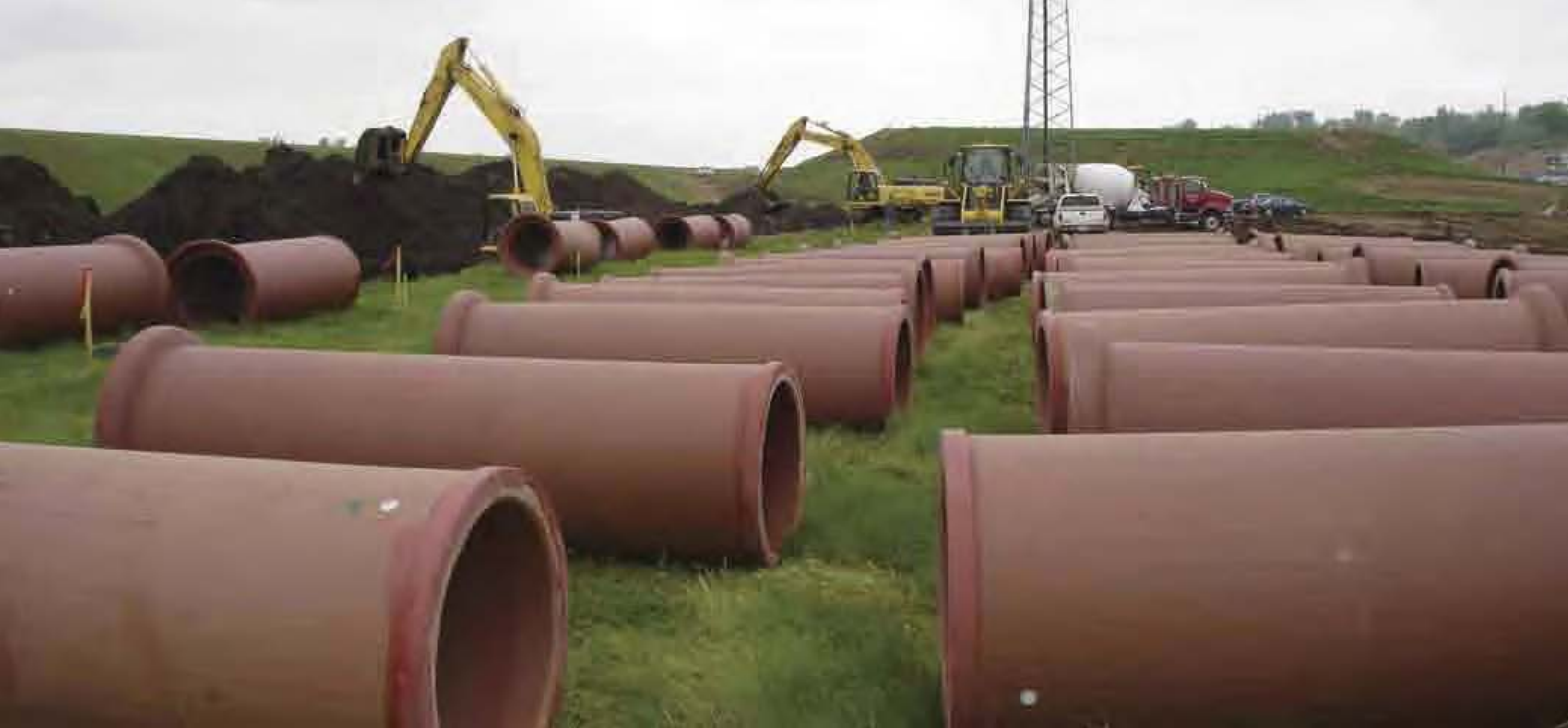
Above: 36-inch Bell and Spigot VCP (10 ft. joints), Sioux City, IA
