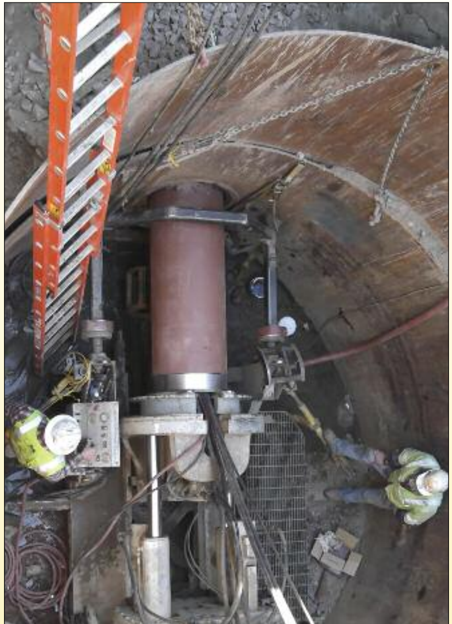
Installing 21-inch pipe in the final phase of the installation
