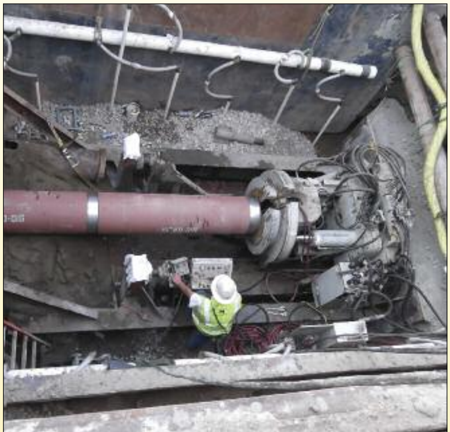
12-by-18-foot rectangular jacking shaft installing 15-inch pipe
