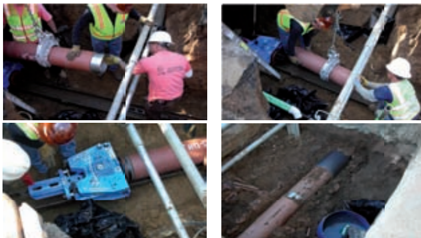
Clockwise from top left: manoeuvring, inserting, pull-through and bursting
