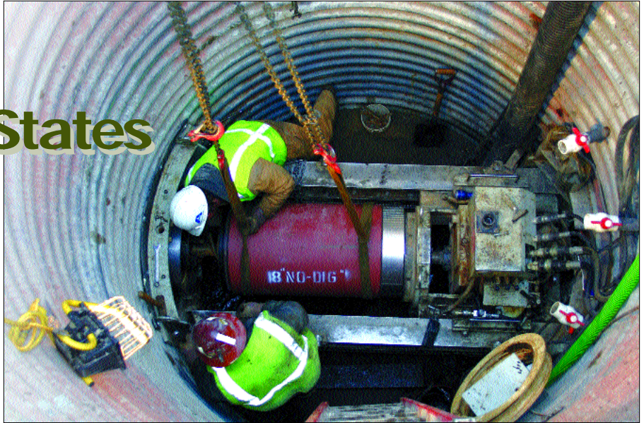
Pilot tube microtunneling has been increasing in popularity in the United States since first introduced in 1995. The method originated in Europe nearly 20 years ago.
