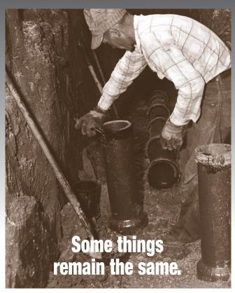
Clay is still the longest lasting, best value product for gravity sanitary sewers. It has always been chemically inert and environmentally friendly.
