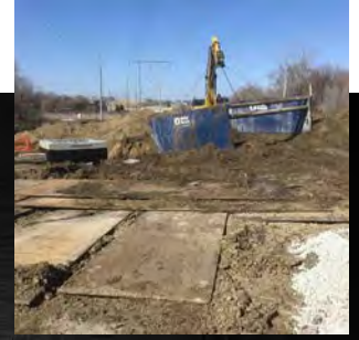
Member's Jobs: L.G. Roloff Construction Company
