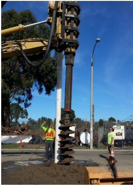
Figure 5: Over 250 wells were drilled at depths ranging from 35 to 40 feet.
