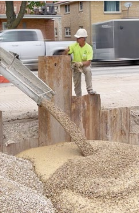
Given the high-traffic surroundings and the need for quick restoration, the backfill method of choice for the shafts consisted of a sand/gravel slurry mix
